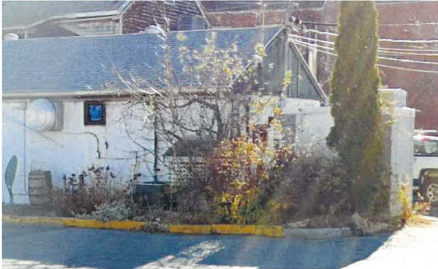
Back End /Walk In Cooler & Utilities
