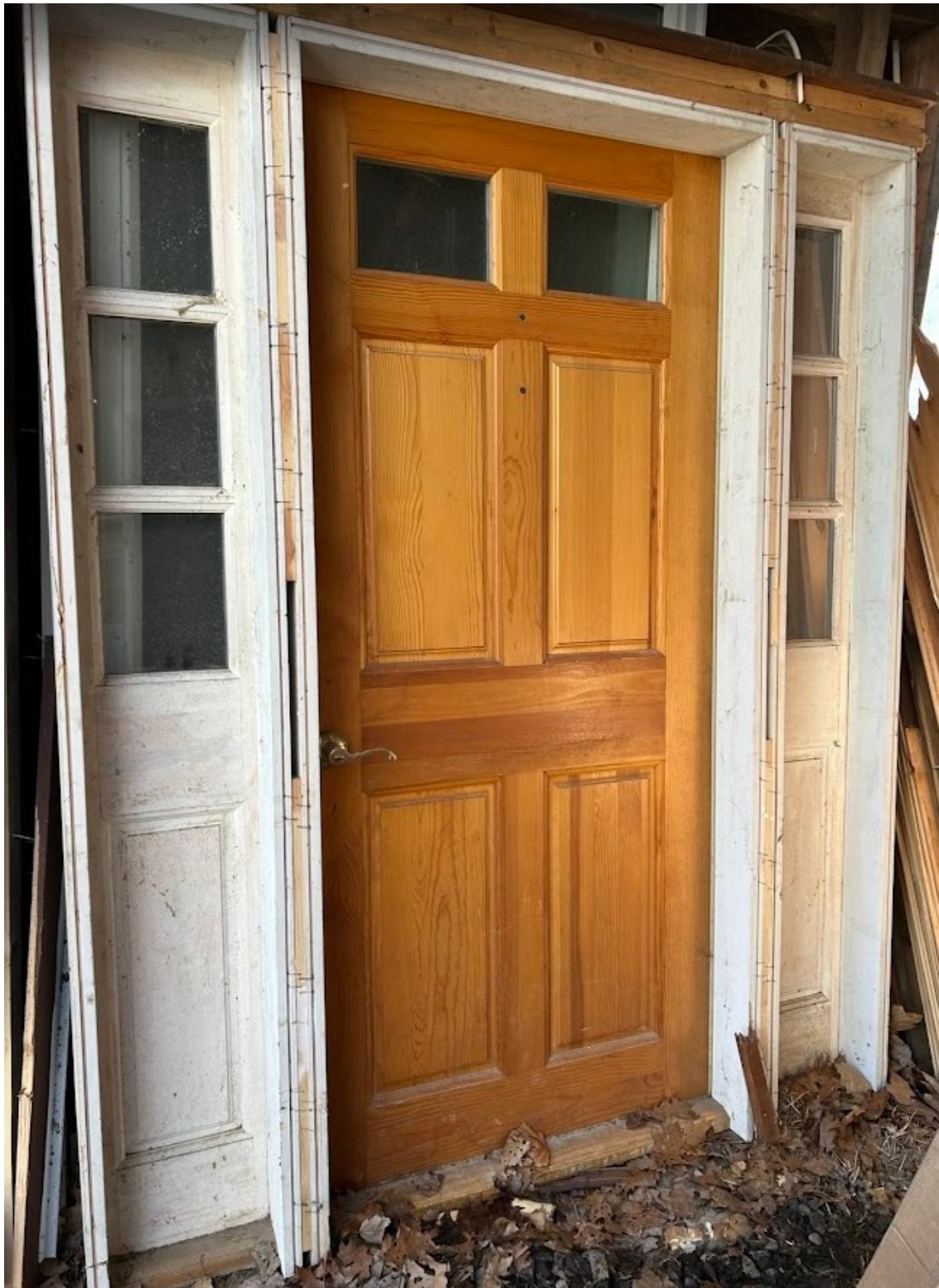
Figure 15: 36" Entry door – wood, with sidelights
