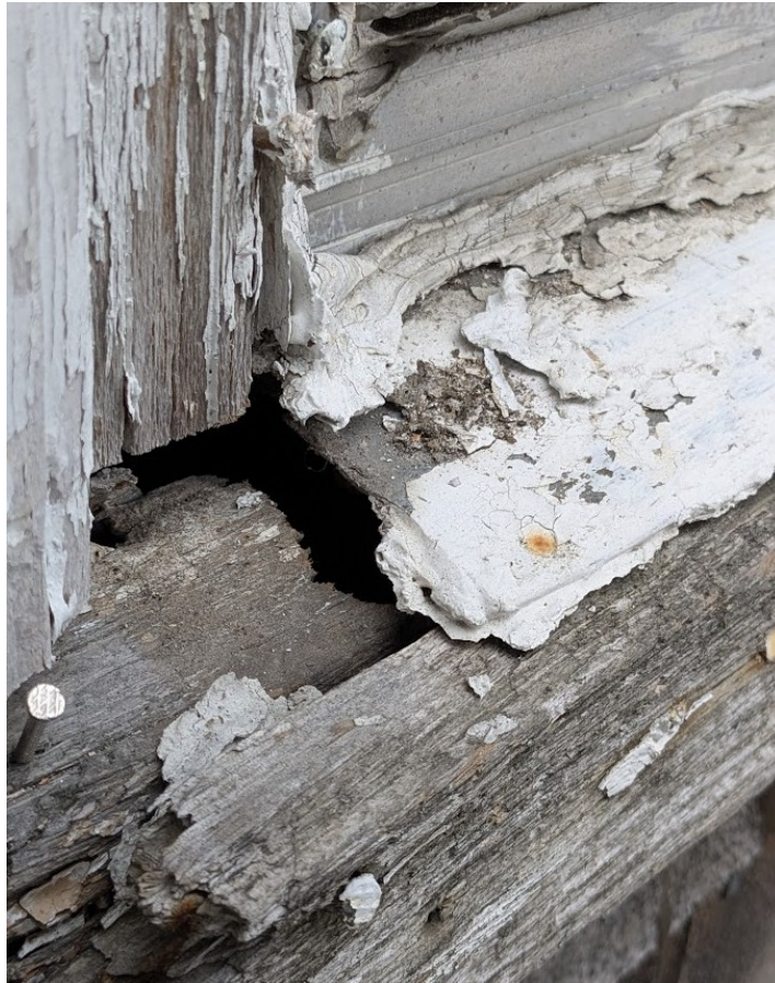
Figure 5: Window sill has rotted away under storm window flashing
