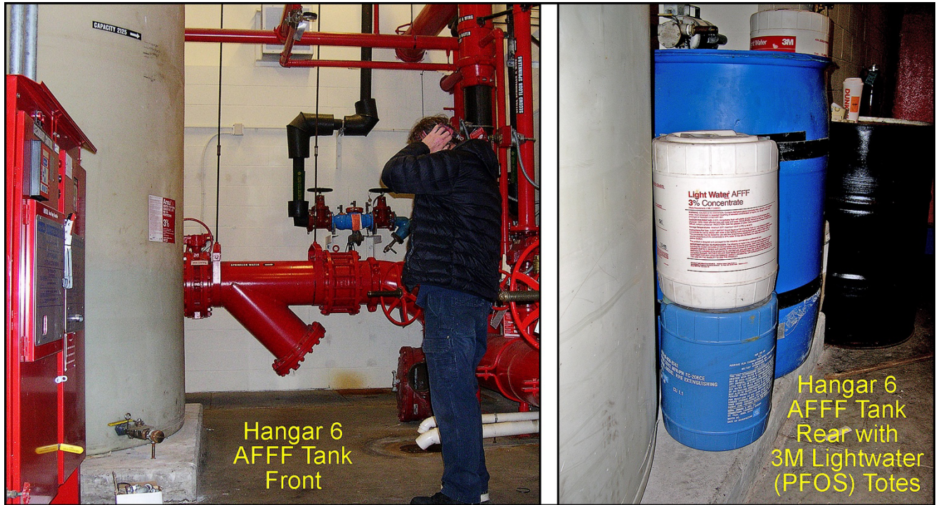
Figure 3. 3M PFOS-based Light water PFOS-based AFFF containers in Hangar 6 AFFF tank room; 11/2023.
