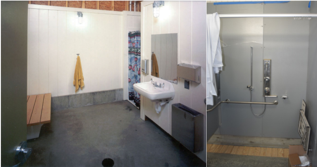
Sealed concrete floors, lavatory, shower fittings, and toilet accessories selected for wet environment and seasonal (non-heated construction)
