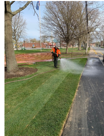
Installation and Watering of New Sod
